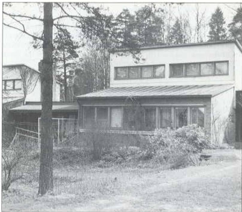
Housing development affectionately known as Kanakopit (Chicken coops), designed by architect Aulis Blomstedt . Photo: Seppo Karusuo.
